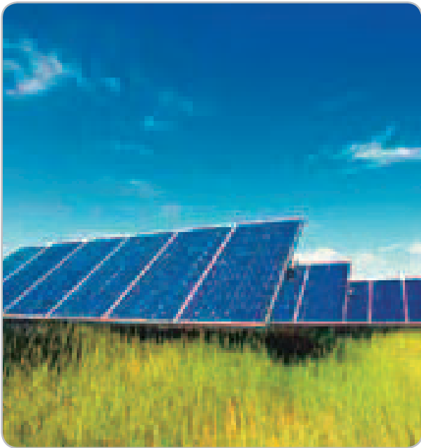
AN EXAMPLE OF A SOLAR FARM IN CALIFORNIA. SOURCE: PROMETHEUS.ORG
