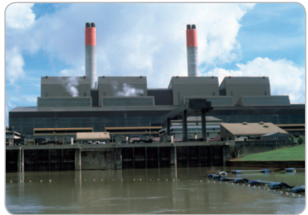
HUNTLY POWER STATION IN THE NORTH ISLAND SUPPLIES UP TO 20% OF NEW ZEALAND'S ELECTRICITY. SOURCE: GENESIS ENERGY
